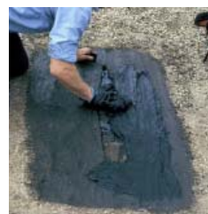
PRIOR TO REPAIRS
