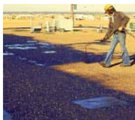
PRIOR TO COATING
